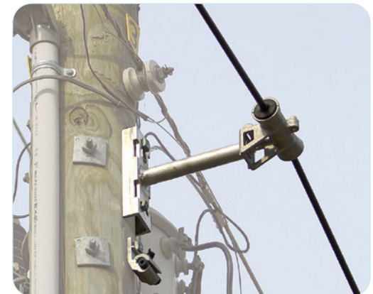
Standoff Bracket with AFL ATGN Single Trunnion
