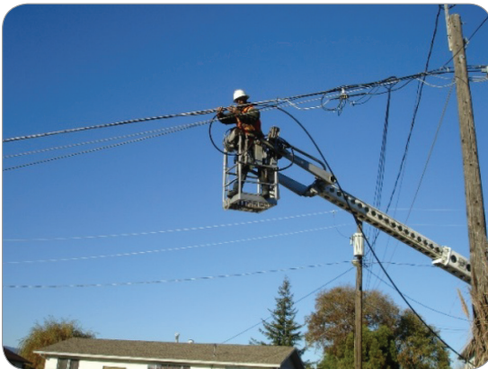
Photograph 9—Aerial 288F WTC Mid Cable Access Point Coil
