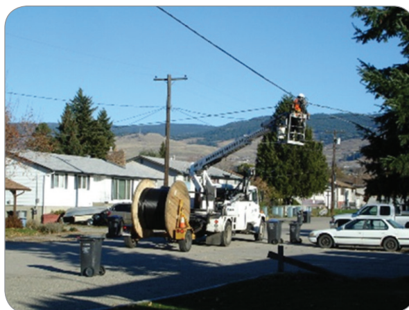
Photograph 2—Aerial Moving Reel Lasher
