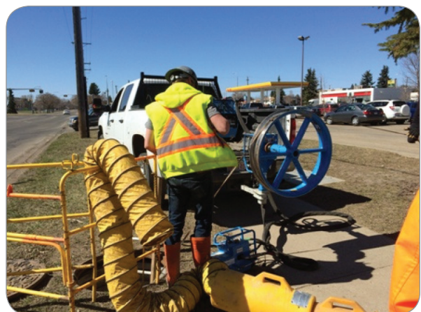
Photograph 1—Underground Puller
