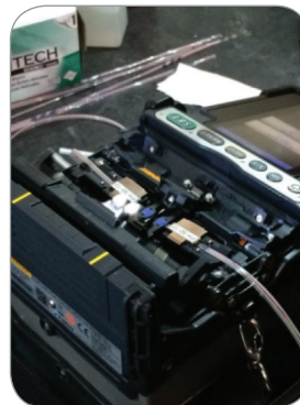
Photograph 15—Mass Fusion Splicing of SWR
