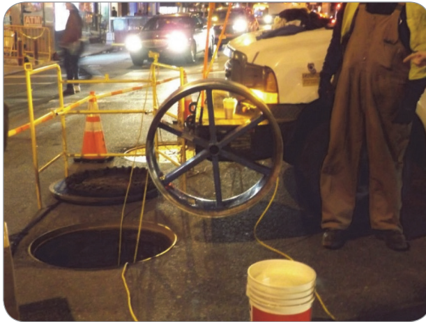
Standard Installation Apparatus Pulling 1,728F WTC
