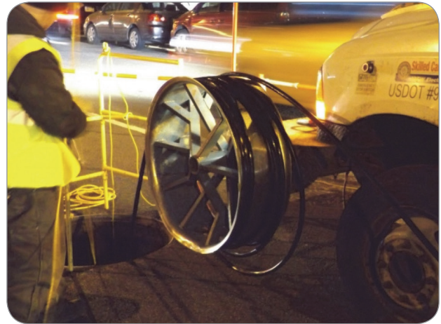
Standard Installation Apparatus Pulling 1,728F WTC
