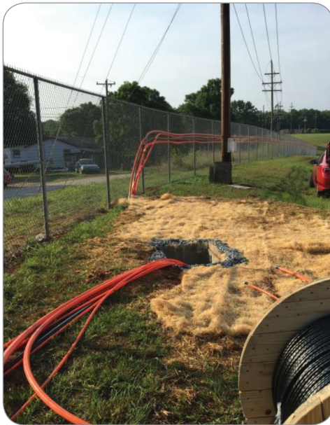
Figure 11—Installation Test Track
