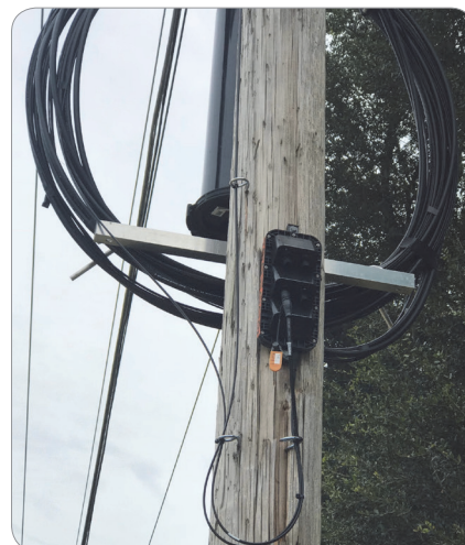
Figure 4—Hardened Pre-terminated Multiport Terminal
