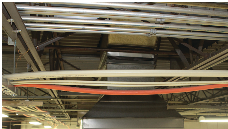
Fig. 6—In this installation example, the eABF riser-rated FuturePath (ivory cable) shows almost no sag whereas the other riser-rated MTC shows significant sag. (Both ducts were installed at the same time and have been in place for over two years.)
