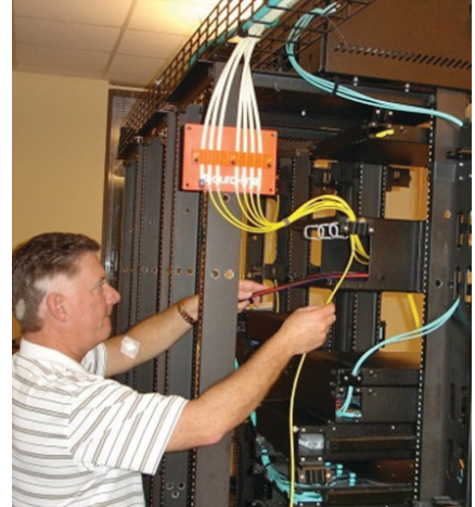
Fig. 5—No furcation tube required to route eABF in cable management space
