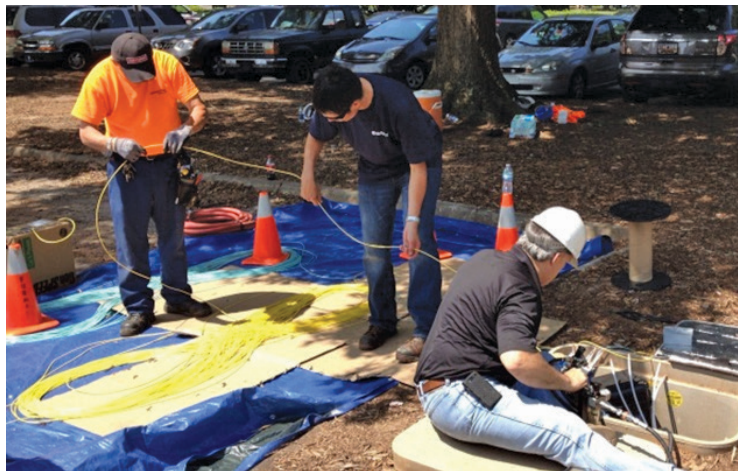
Fig. 4—Mid-span figure 8 using onward blow method. With this installation technique, eABF cable can be installed over great distances.
