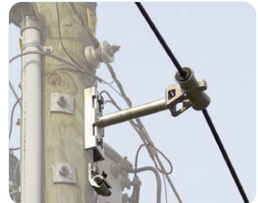
Standoff Bracket with AFL ATGN Single Trunnion
