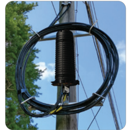
Coil Bracket holds excess ADSS cable
