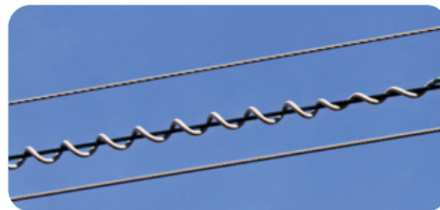
Spiral Vibration Damper on ADSS Cable
