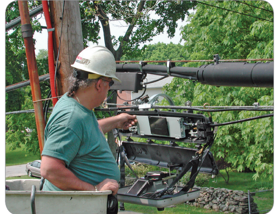
Installation of a Weather-Tight Aerial Splice Closure
