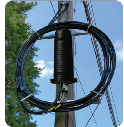
Coil Bracket holds excess ADSS cable
